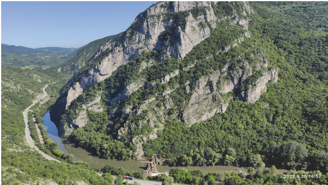
Hydroelectric power plant “Sveta Petka” located in the Sićevo gorge (Designed by Nikola Tesla and Djordje Stanojević)
